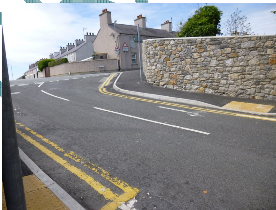
Photograph 9 – New Footway link from Gwynfa Hill to Mill Bank
