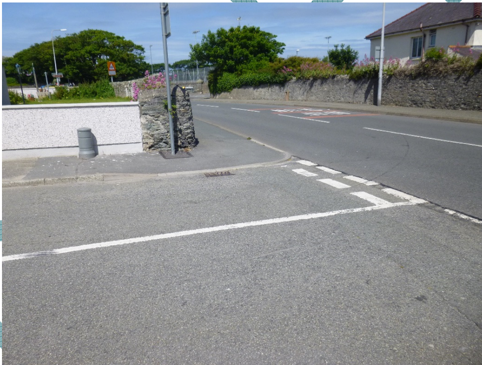
Photograph 17 - Drainage Gully in Line with Crossing at Maes Cybi (north)
