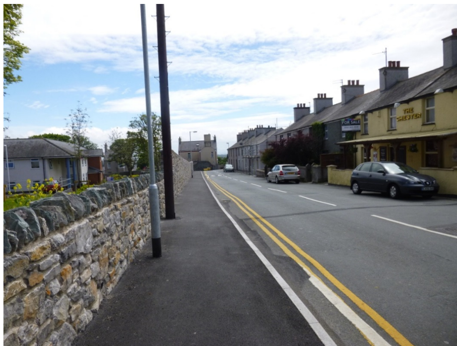
Photograph 8 – New Footway along Mill Bank
